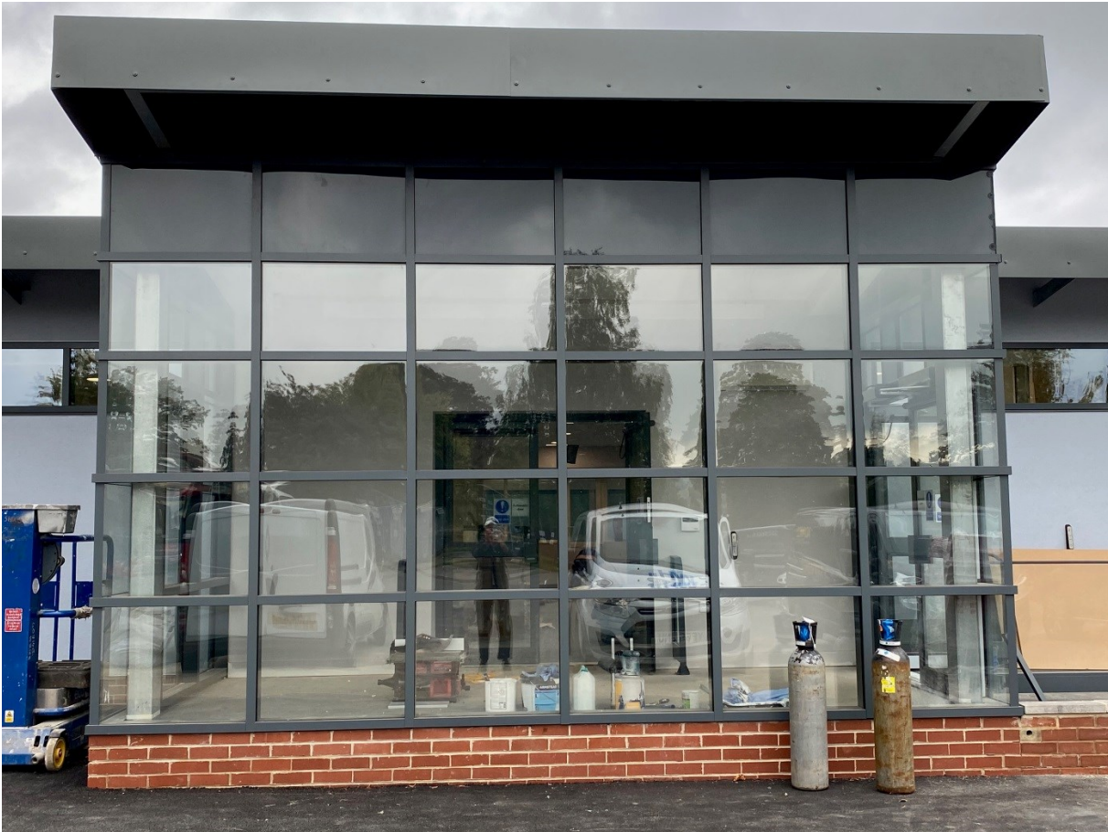
The entrance hall takes shape. Summer 2022
