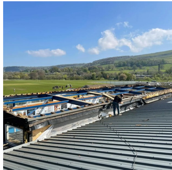
Up on the roof
