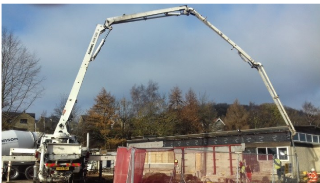
It's a big job putting in the foundations
