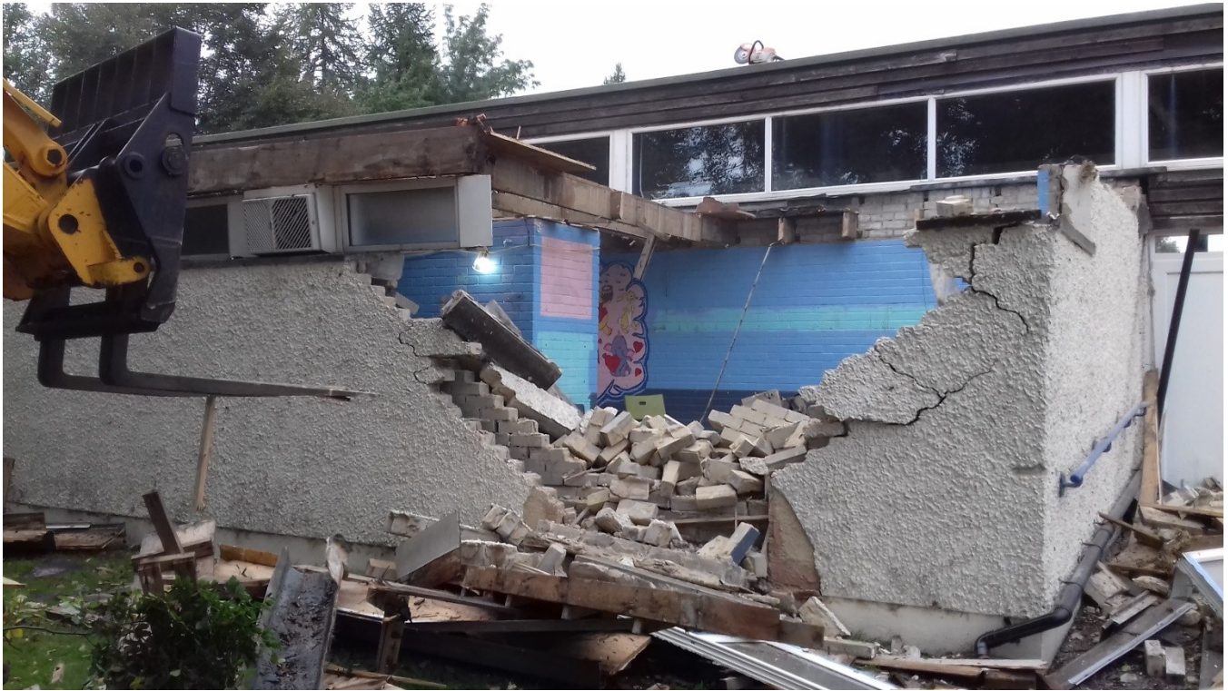
October 2021 - the bulldozers move in
