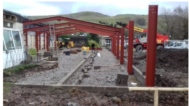
The new build starts to take shape
